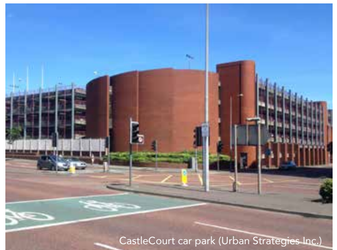
Car parks on the unfinished South Link of the Inner Ring Road (Urban Strategies Inc.)
