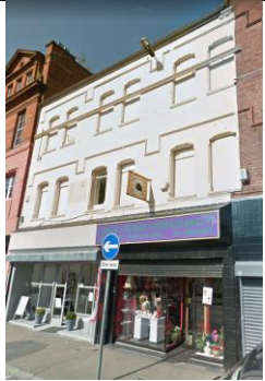
29A-31 NORTH STREET (ST. ANNE'S BUILDINGS)
